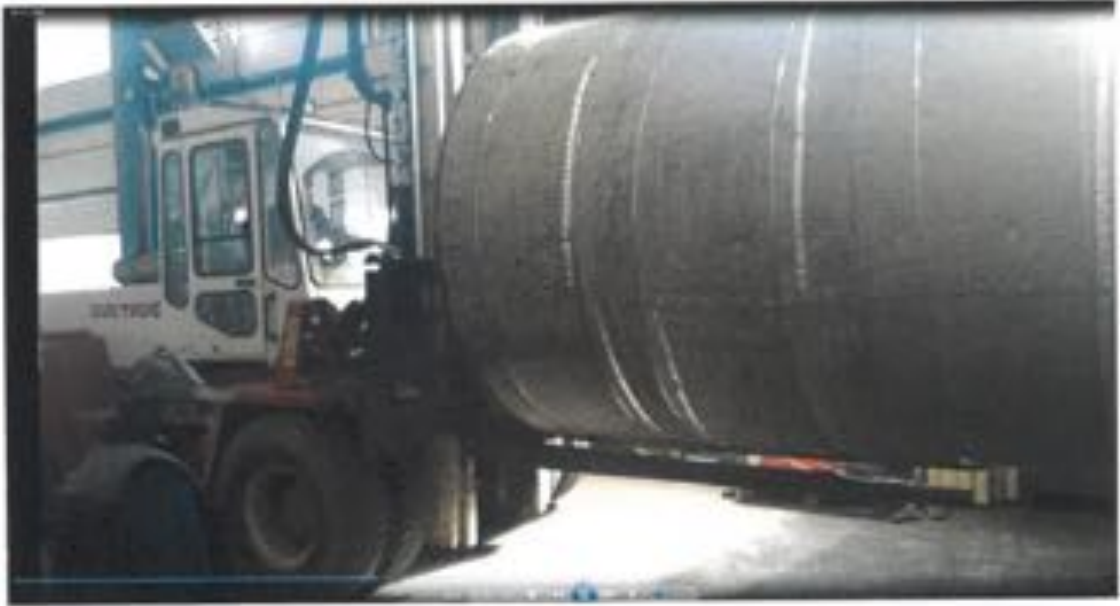
Photo of chimney insulation during assembly in Košice
