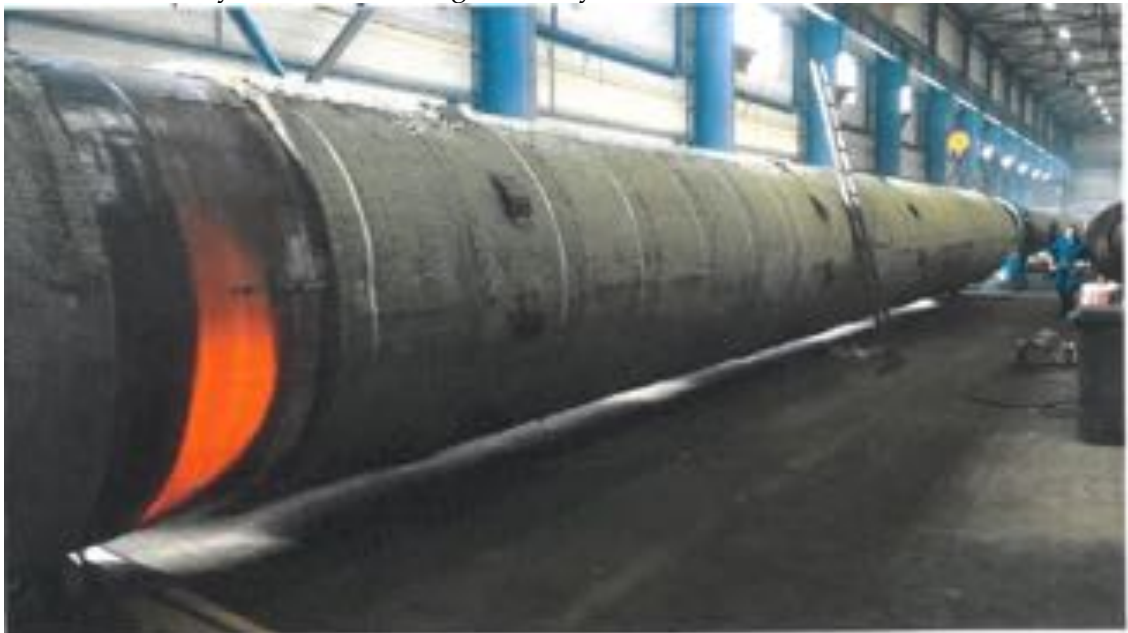
Photo documentation of insulation damage dated 10.10.2018
